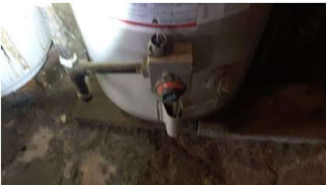
13.17 Water Heater Condition:
