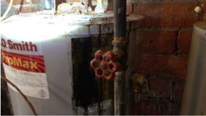
13.15 Temperature & Pressure Relief Valve: Serviceable
