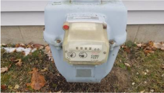
Gas Line Primary Piping Material: Black Iron Pipe.
